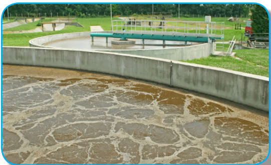
Waste Water Treatment
